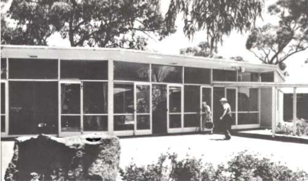
The community centre at the Carrum Downs village settlement for elderly people. Australian News and Information Bureau
