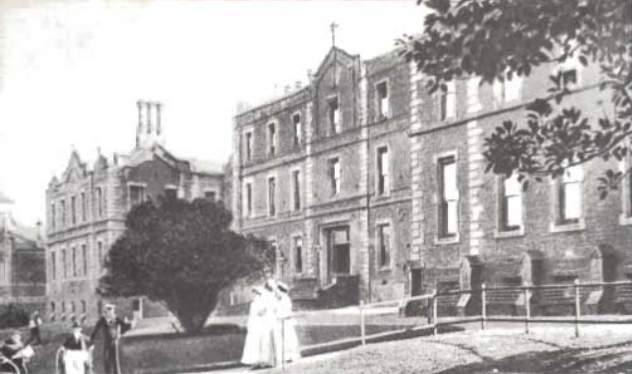
The former Royal Melbourne Hospital building in Lansdale Street, now the Queen Victoria Hospital
