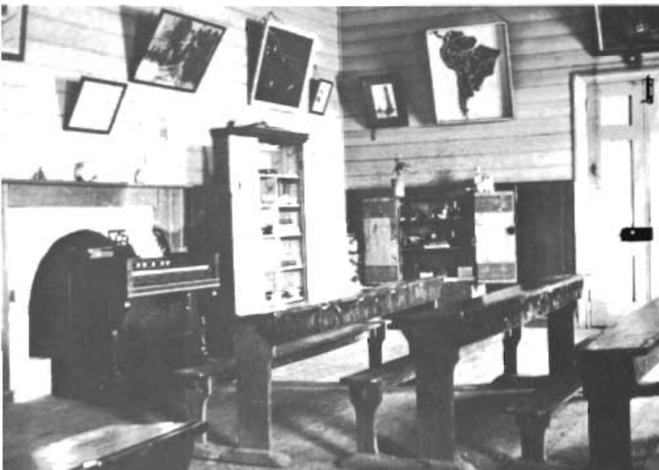
Interior of an early primary school. Education Department
